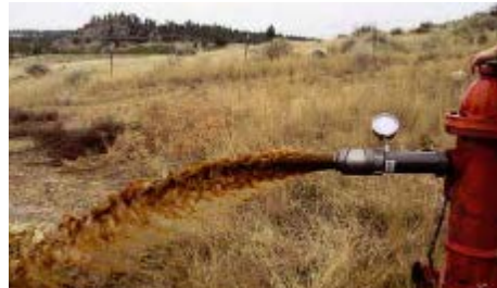
A recent hydrant flushing shows the quality of water in Roundup, Montana. The City currently provides disinfection as a sole source of treatment. Disinfection is provided by chlorine gas.(CMWRA 2014 Appendix 8: Appraisal Report page 12).
